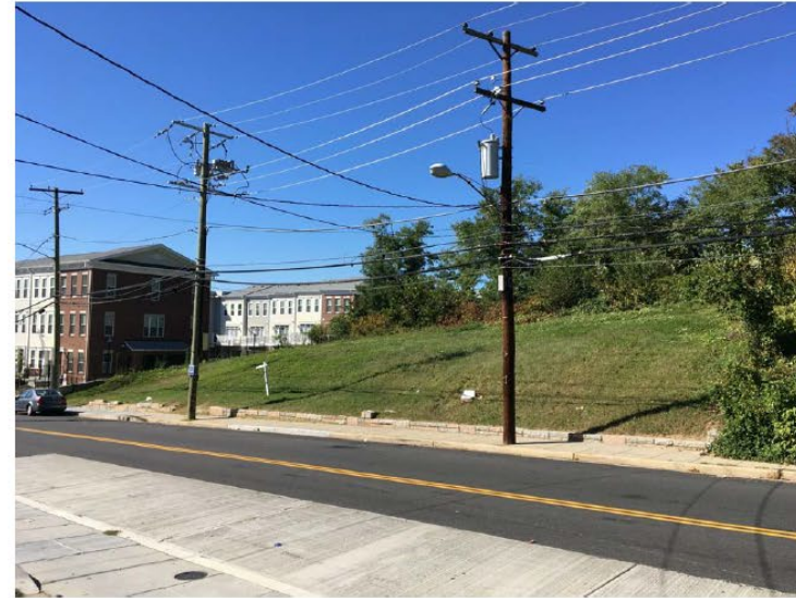
SITE FROM SE
